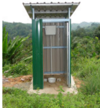
The old pit latrine behind the kindergarden and the new flush toilet at Kg. Lapan..
